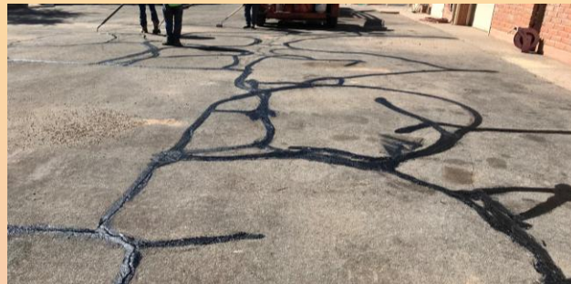
Crack seal Coronado National Memorial
