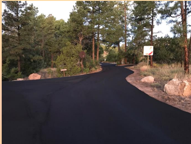
Micro surfacing in Juniper campground C-loop.
